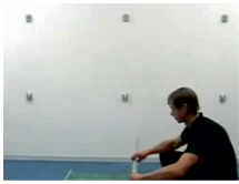
Fitting of the wall mountings.
