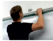
Insert the lock-in rail in the upper wall bracket and lock in place.
