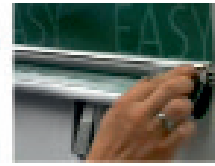
Insert the lock-in rail in the bottom keder profile and lock it in place, too.
