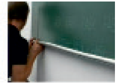
By pressing the keder profiles up or down, the fabric is tensioned.
